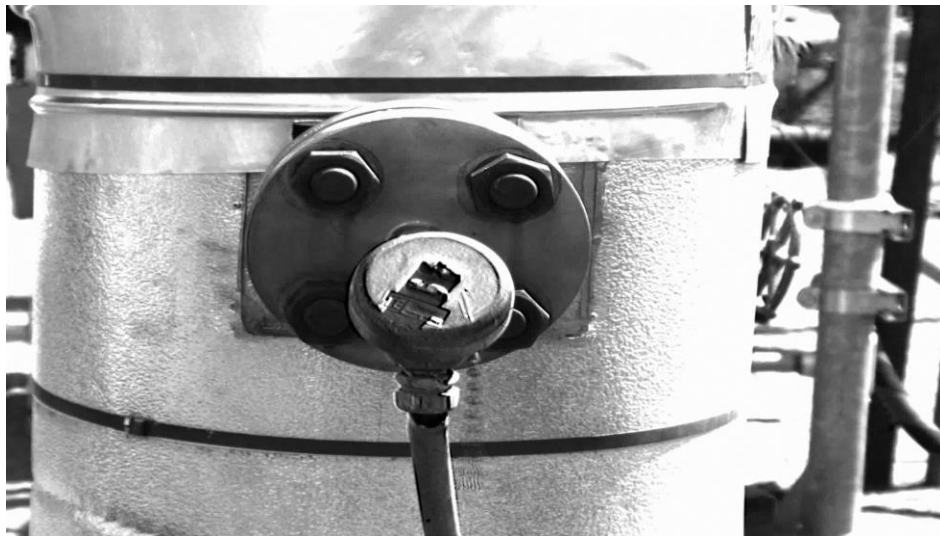
Figure 5: Frame of the MAV process applied to a gas pipeline small bore thermowell
